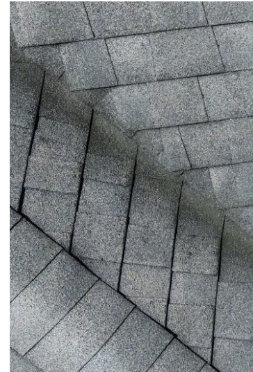
Representative granule loss at valley
