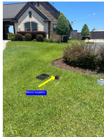
Water meter location - right of driveway near street
